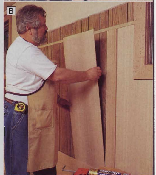
Align the mullions, as in Photo A , to check your layout. The inset shows how to hold them before you're ready to nail. Slide the panels into place, as in Photo B . Fit the window trim pieces, as in Photos C and D .
